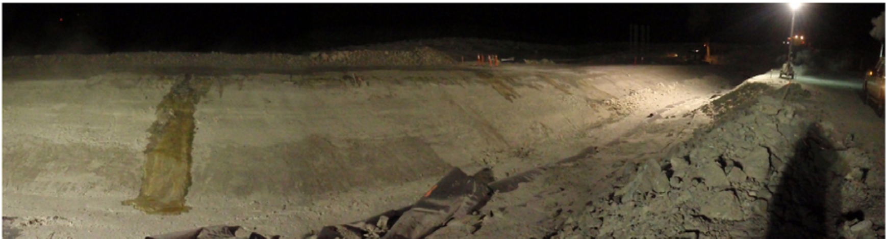
Photo 14: ~NNE stitched panoramic view of upstream dam slope. Taken from around 1+20 Note the ice on the slope around station 1+15 is expected to be scraped back when the next lift is placed in this area. Ice from water discharge down slope, due to water draining to a low graded point in the placement.
