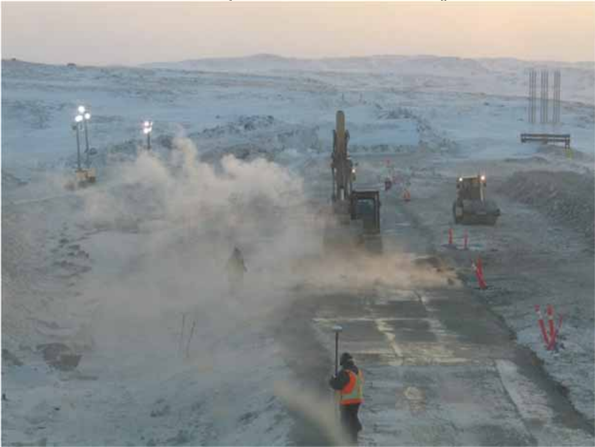
Photo 3: Surveyor taking as built measurements at the end of the shift
