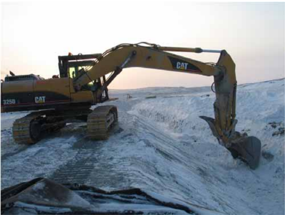
Photo 9: Excavator cleaning snow in berm key trench
