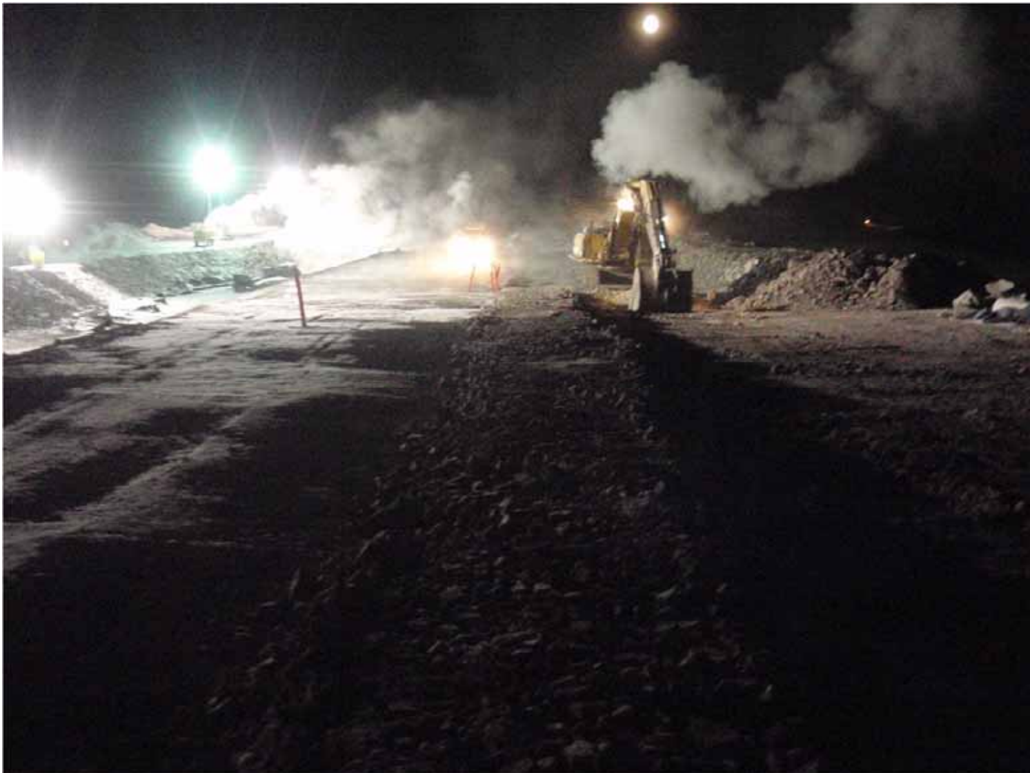
Photo 14: ~330 Excavator placing Transition material along downstream edge of FCM placed today.
