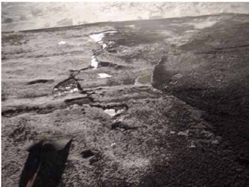
Photo 10: Slight cracking on top of dayshift placement near tie in. This area is planned to be revisited after freezeback.
