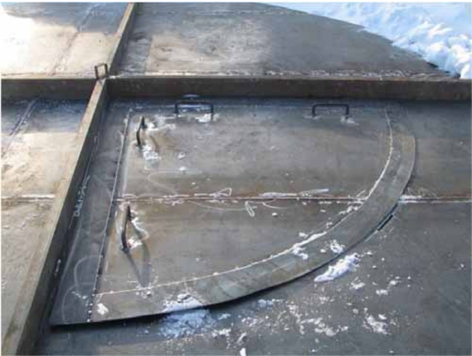
Photo 5: Section cut out to install sumps
