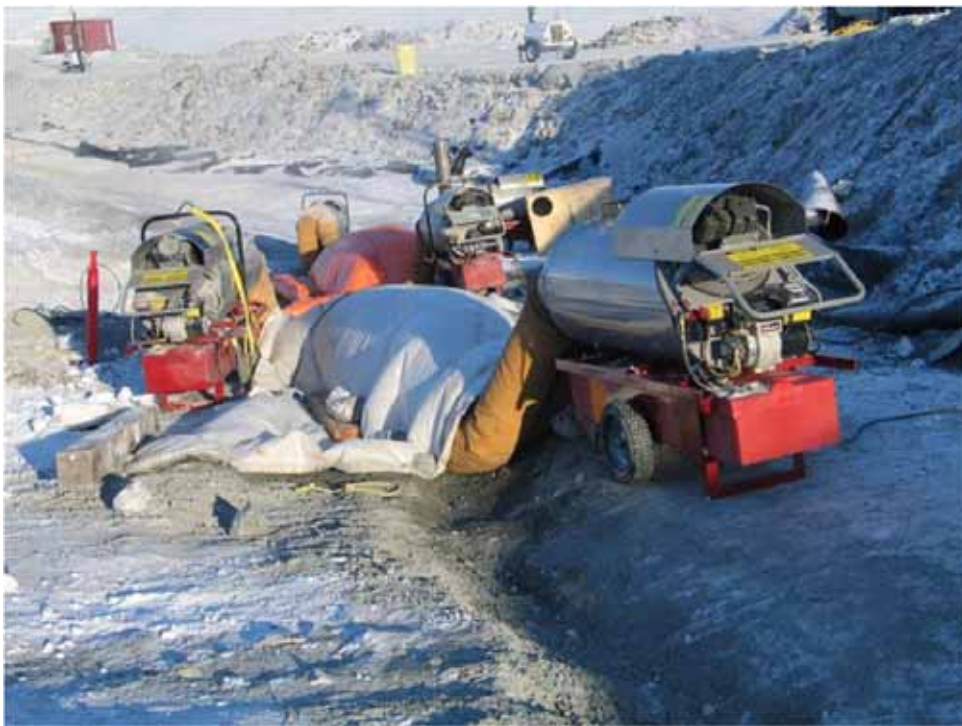
Photo 8: Frost fighters heating and hording around the fillet expansion around 0+70.
