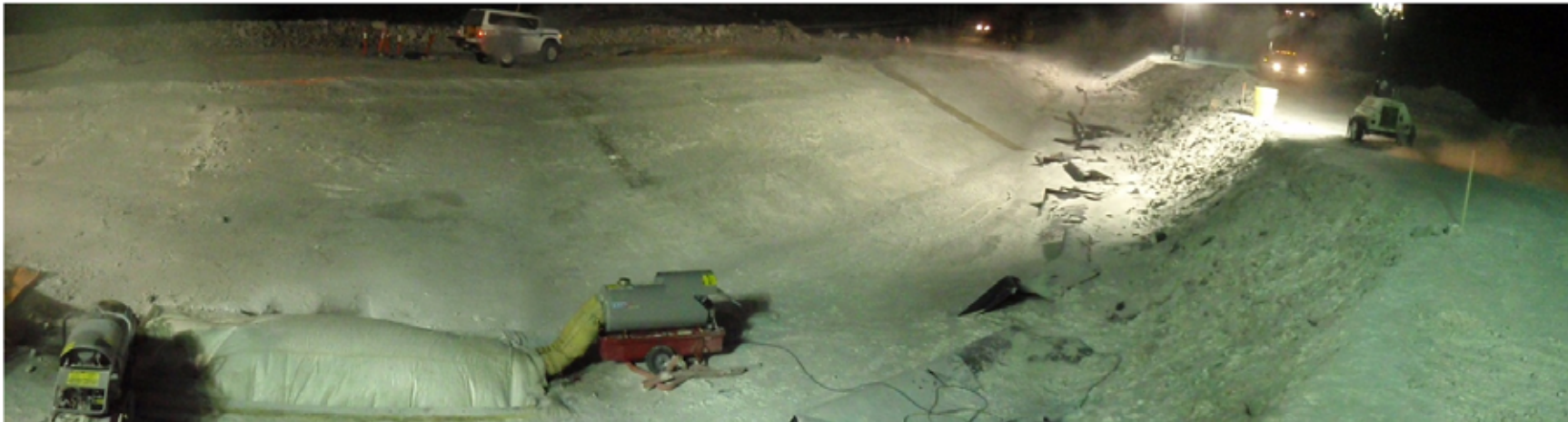
Photo 14: ~WNW view of the upstream dam slope. Taken from around station 0+75. Note the hording and heating being completed around 0+70 .
