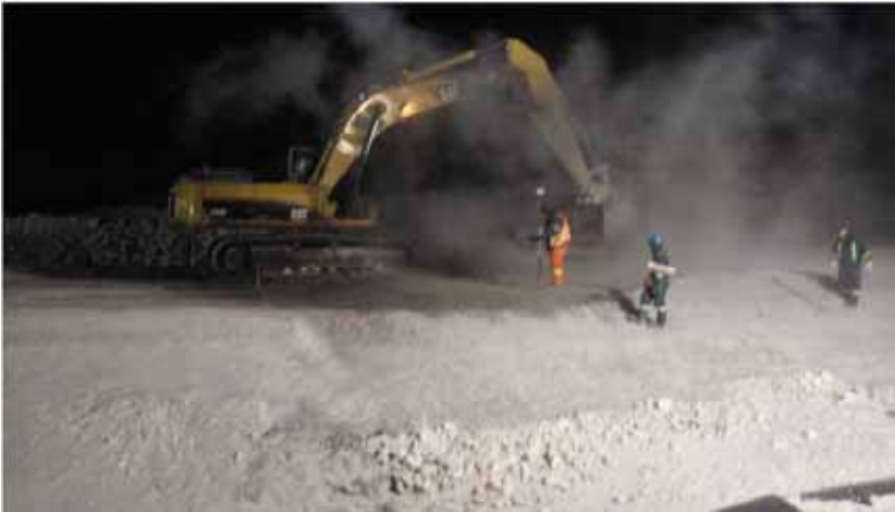
Photo 12: ~N view of construction crew working on sloping upstream of dam.
