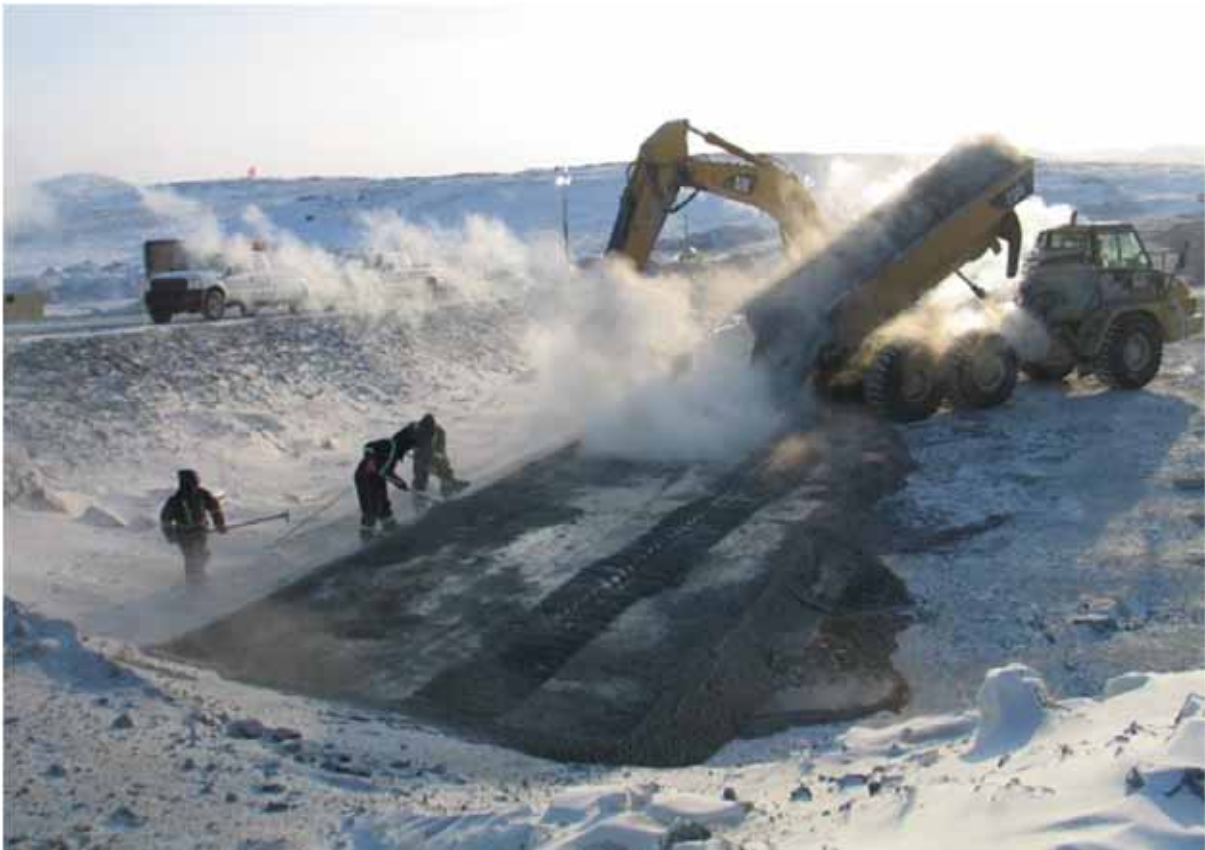
Photo 2: Placing core material at extreme north end of the key trench. This section is now at final grade.
